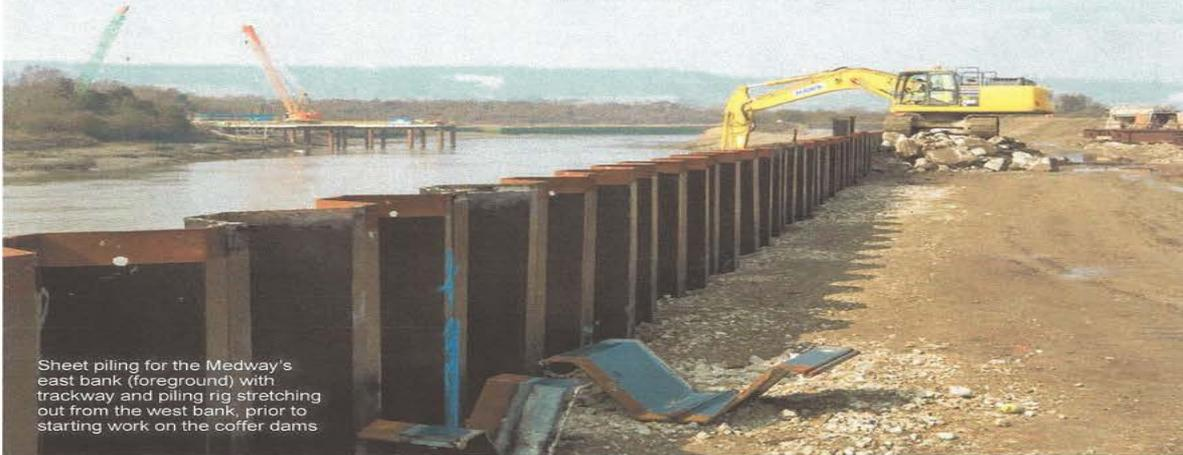
Sheet piling for the Medway's east bank (foreground) with trackway and piling rig stretching out from the west bank, prior to starting work on the coffer dams
